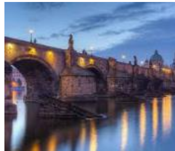
Charles bridge - Prague
