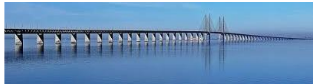
Øresund bridge – Denmark – Sweden
